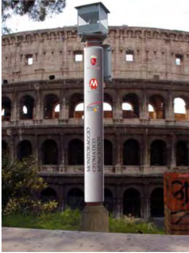
Fig.4 Total station for monitoring
