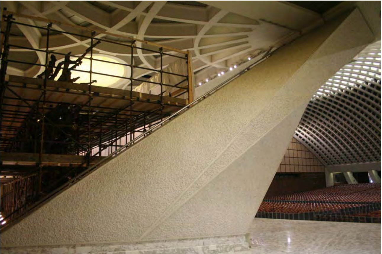
Fig. 17: The restoration shipyard.
