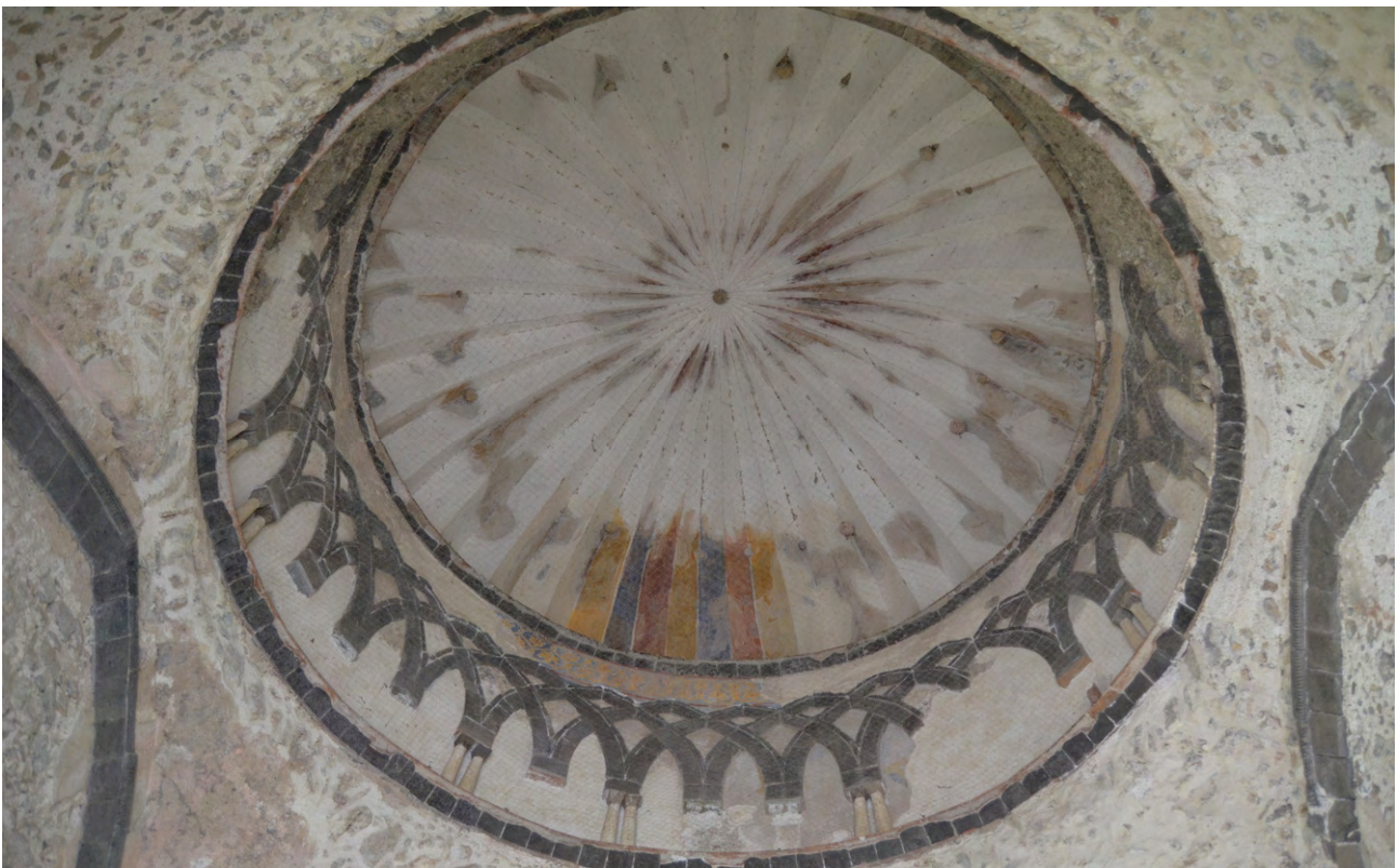
Fig. 1: Ravello, villa Rufolo. The dome of the entry tower shows various Islamic influences
