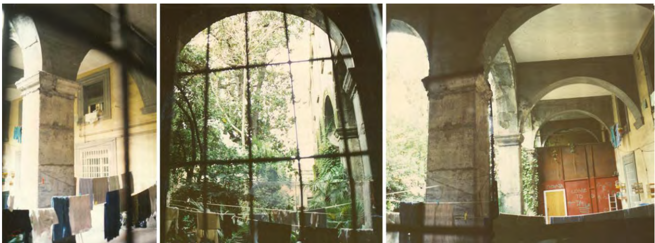
Illustration 8: The current state of the arcade of cloister.
