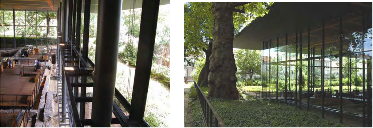
Fig. 7, 8: Périgueux, domus de Vésone, partial internal and external view of the protective structure.
