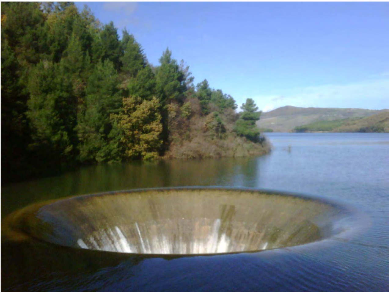
Fig. 1: View of an overflow in full-water condition.
