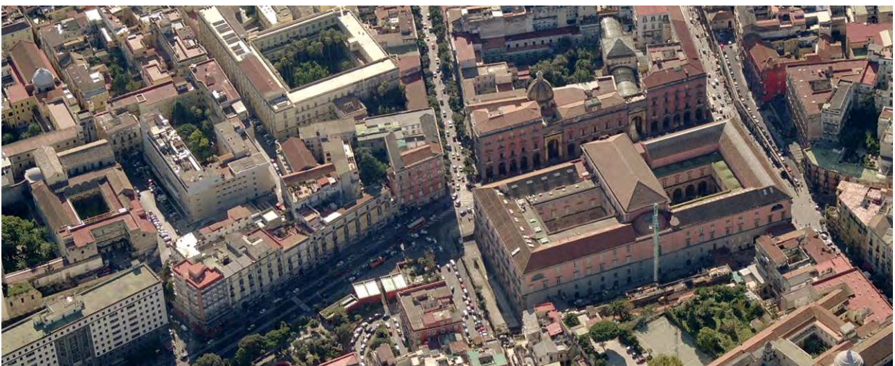
Illustration 2: Close aerial image of the urban context of S. Aniello a Caponapoli.
