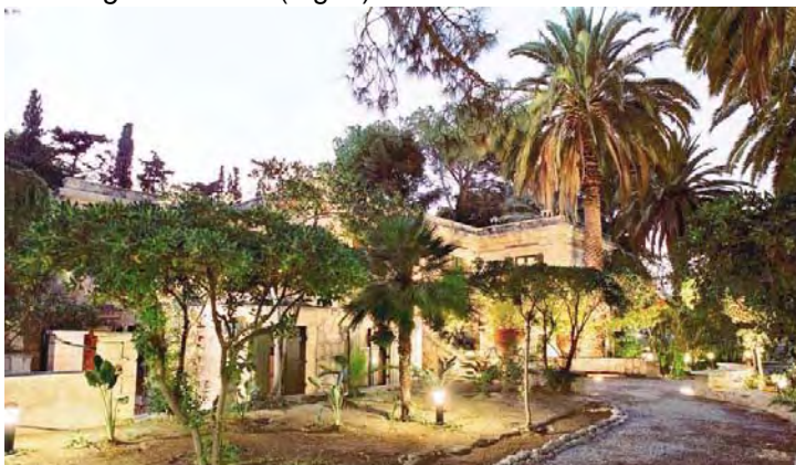
Fig. 3: View from South - East of main façade of Villa "Ariadne", 2004.
