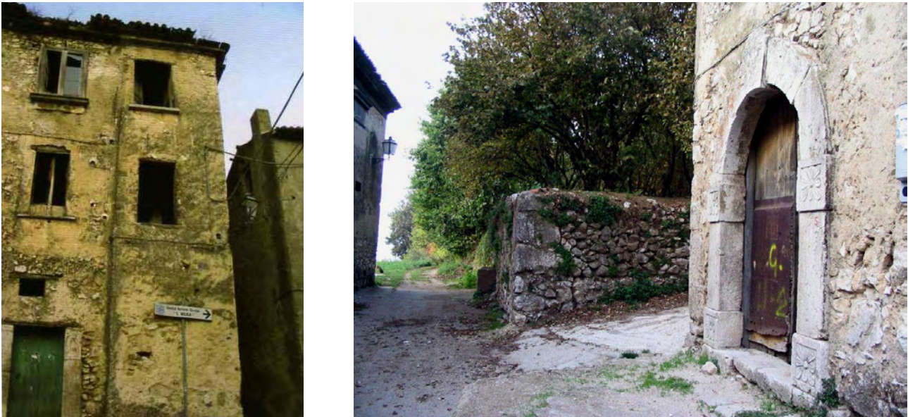
Fig. 3: Casale Castello - Defense building types: the tower-houses
