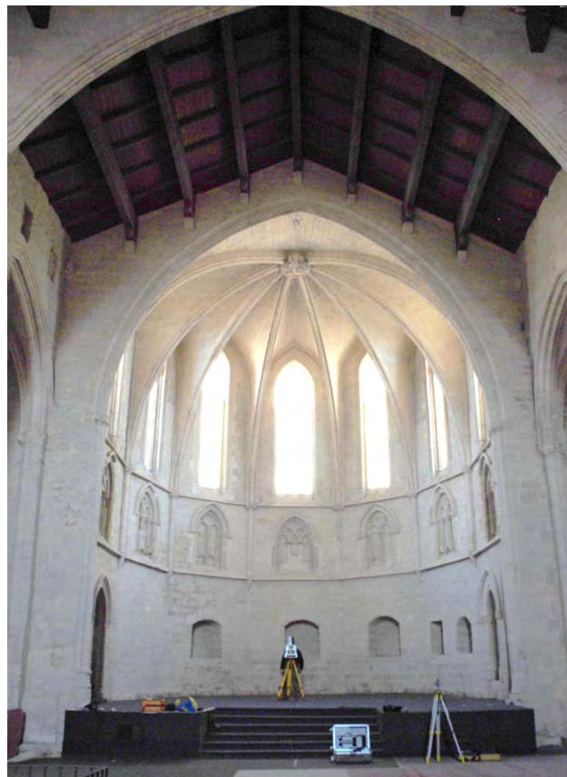
Fig. 1: General view of the apse of the Church of San Francisco
