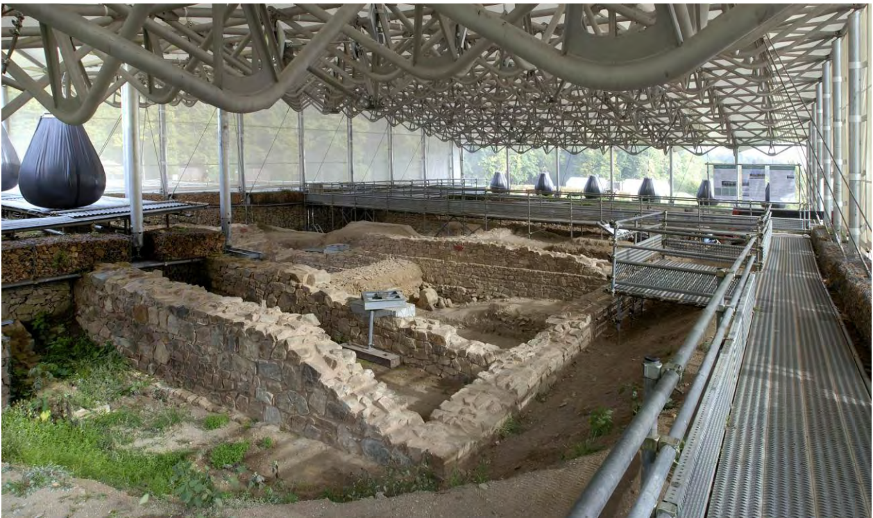
Fig. 10: The shelter designed to protect an area of architectural remains of major importance – those of a mid-1 st c. BC forum – built without foundation and made of a frame whose pieces weigh only 42 kg each (architect: Paul Andreu ; Antoine Maillier ©Bibracte)
