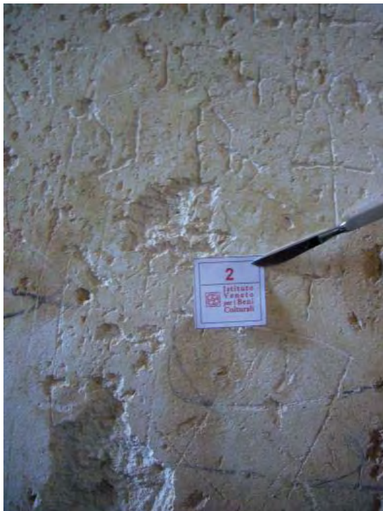
Figure 3. Sampling point 2: finishing plaster placed inside, Ottoman period.
