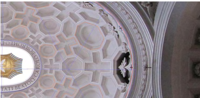
Fig. 1: Photo of the dome (C. Falcolini) and overlay of the photogrammetric restitution and geometric construction of the "canonical oval"
