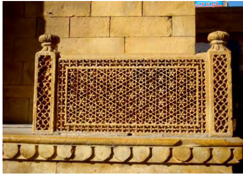
Fig. 7: Number of carved Stone blocks used in jali depends on desired Length and width.
