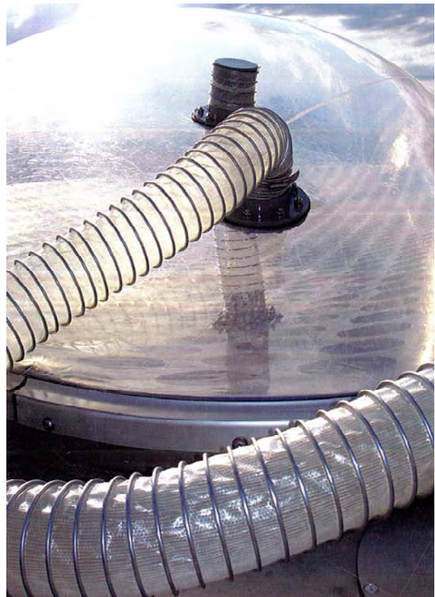
Fig. 14: Detail of the roof 'pillows', showing ducts that regulate solar penetration by inflation and deflation. [29]
