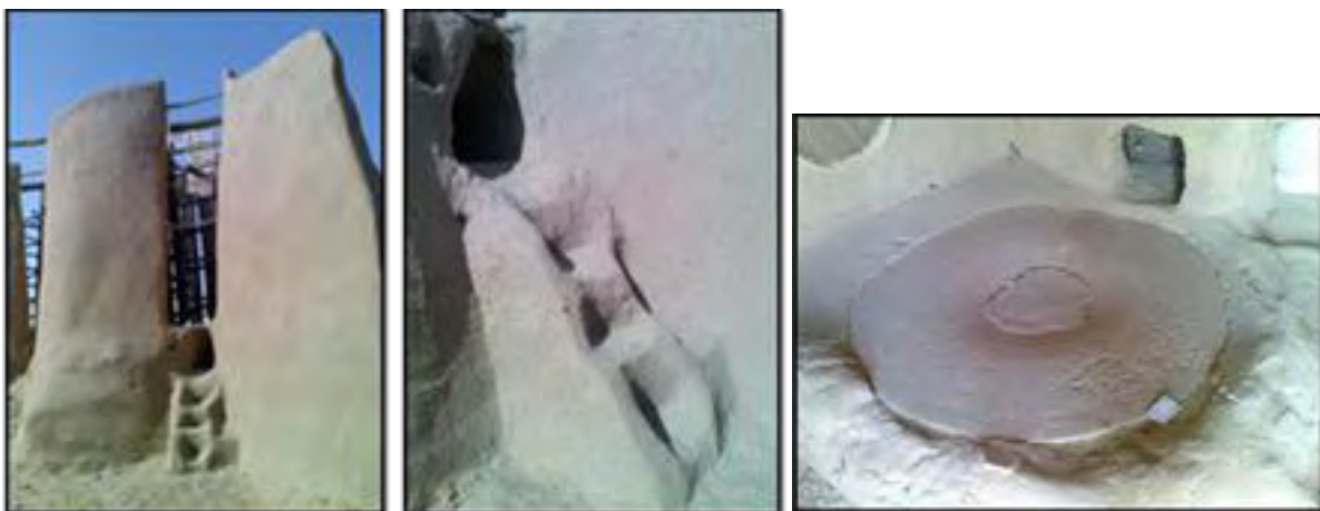
Figure 4. Wind gate position on interior and exterior walls. (Source: Writer)
