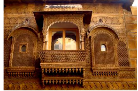
Fig. 8: Stone jali covering the window and window.
