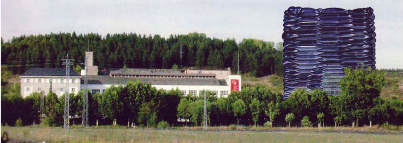
Fig. 16: General view showing the inflatable façade. [34]
