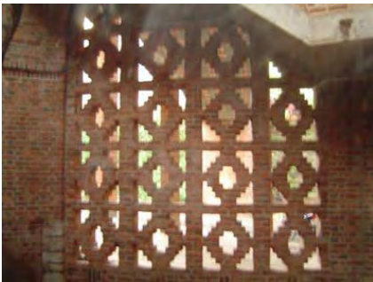
Fig. 13. Laurie Baker's Brick Jali. http://lauriebaker.net/work/work/pictures-of-buildings.html
