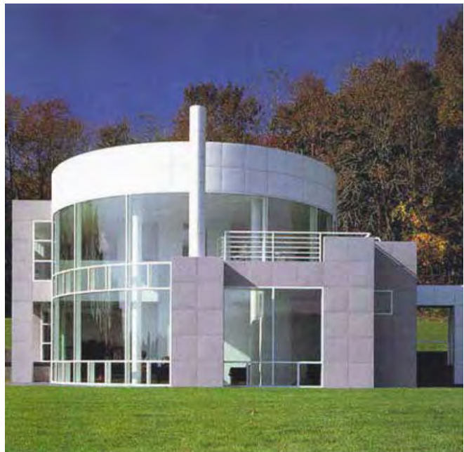
Fig. 14: Grotta House, New Jersey, 1983-89
