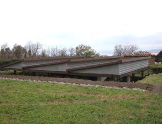
Fig. 15, 16: Stabia, Villa di Arianna, general view of the roof covering the spaces of the H-O-R-S-T-U and detail of the system of fins wrapping the space.
