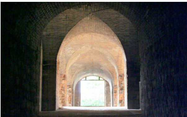
Fig.9: Forte Portuense, vaulted ceiling.
