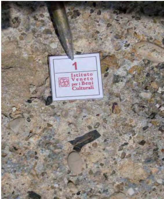
Figure 2. Sampling point 1: bedding plaster placed outside, Crusader period.
