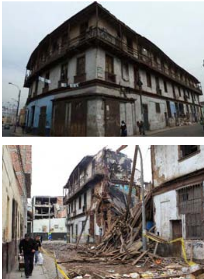
Fig.1-2: Casona El Buque before and after the collapse. In November 2012, a fire caused the collapse of this historic mansion built in 1753 and designated national monument in 1988.
