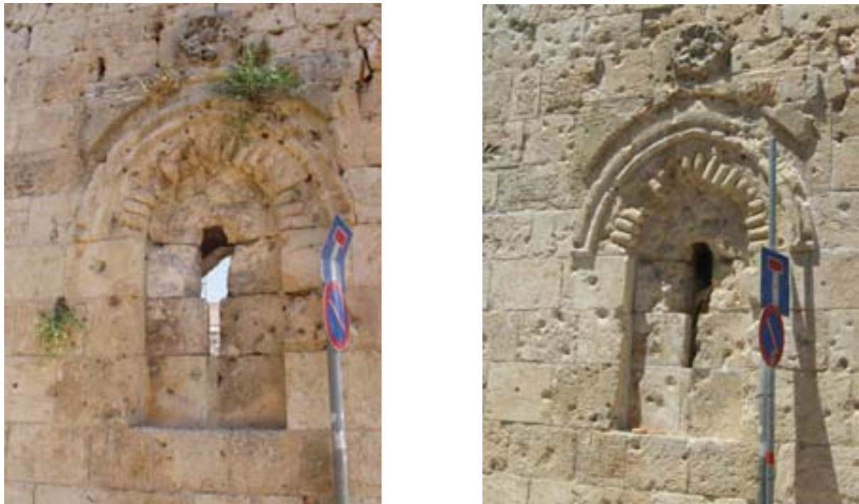
Fig. 5: Stone deterioration and vegetation that took root in an arrow loop, before and after the conservation work.
