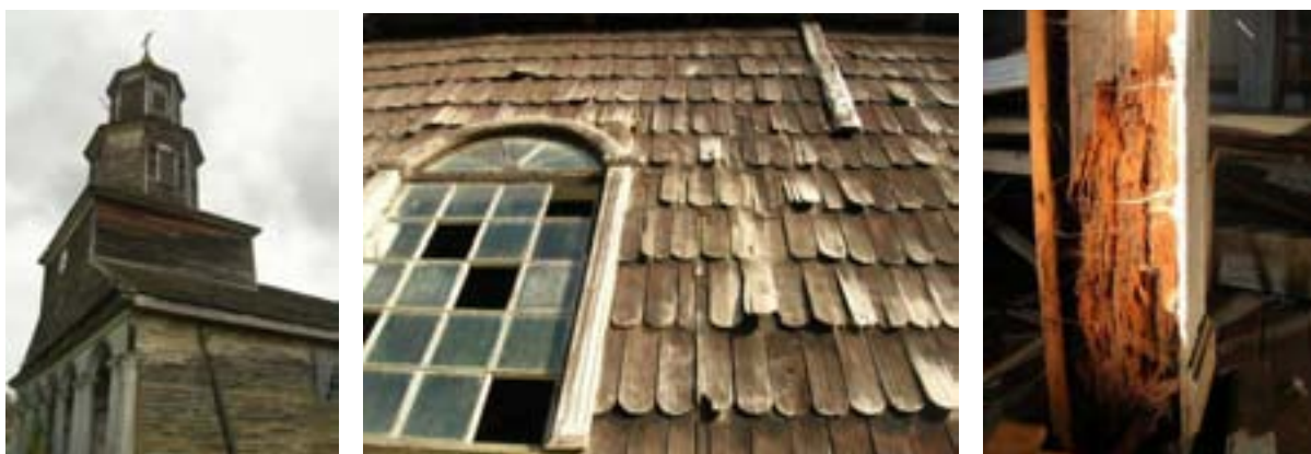
Fig. 3: The decayed elements of a church comprises the exposed surfaces of the wood, to areas usually hidden to the naked eye. The putrefaction of a timber and the presence of wood boring insects can therefore place a serious threat to the stability of a main structural element. (Photographed by the author: churches of Nercón 2009, Rilán 2006, and Quinchao 2006).
