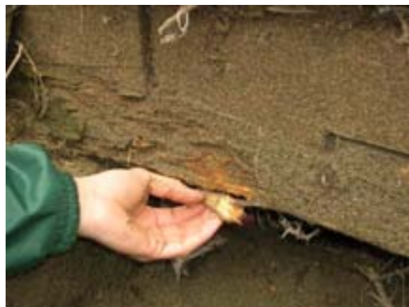
Fig. 7: Vilupulli, before restoration. Climatic factors and the wood boring insects had seriously damaged the structure of the building. (Photographed by the author, 2005).
