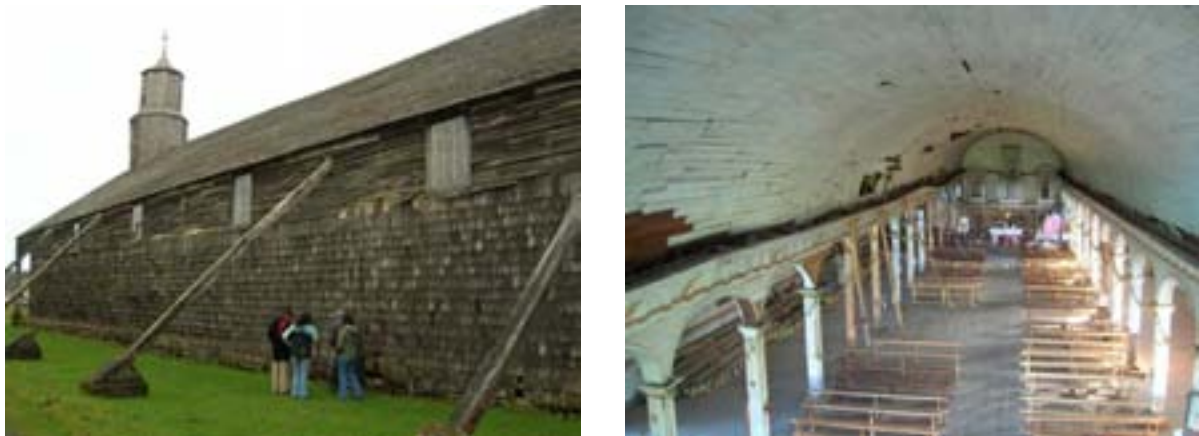
Fig. 2: Quinchao, one of the 16 UNESCO World Heritage wooden churches prior to the 2011 full restoration. Exterior and interior view. The extensive and severe decay of the structure threatened the building to collapse. (Photographed by the author, 2006).
