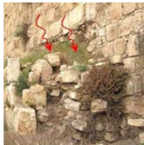
Fig. 3: The seepage points of water into the wall and its further results.
