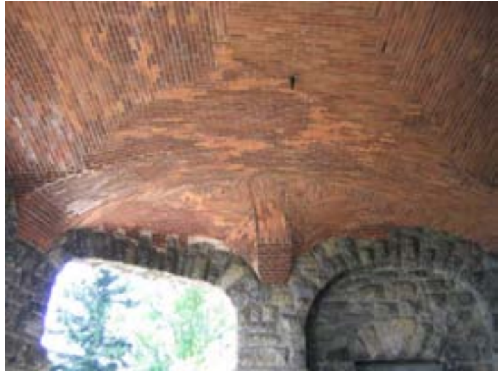
Fig.3: Brickwork vault of the Restaurant at Campo dei Fiori by Giuseppe Sommaruga
