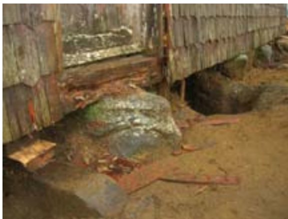
Fig. 7: Vilupulli, before restoration. Climatic factors and the wood boring insects had seriously damaged the structure of the building. (Photographed by the author, 2005).
