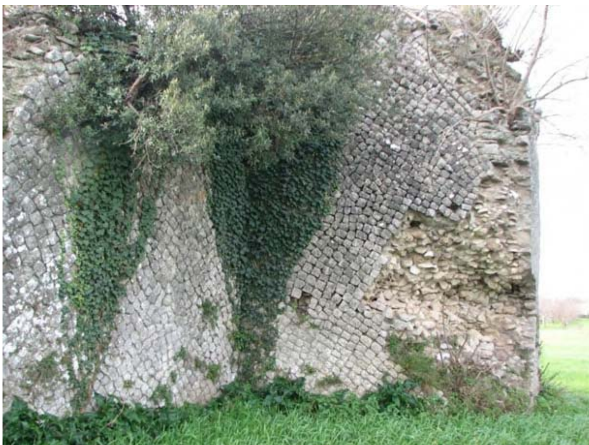
Fig. 2: Detail of insertion hexagonal tower-curtain wall.
