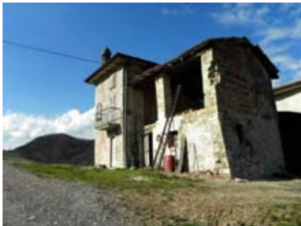
Fig. 7-8: Val Chiarone , district of Pianello Val Tidone , Piacenza . At left: La Costa – “the shore” –, rural building characterized by stone masonry and clay tiles roofing; next to the house there is the stable and, over it, the hayloft. At right: the Casotto with its dovecote tower and the surrounding landscape; it is evident the position of the compound in relation to the hill (photos by Valentina Cinieri, 2013).
